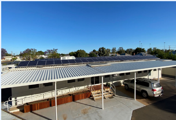
Solar panels on the Council Chambers roof.
