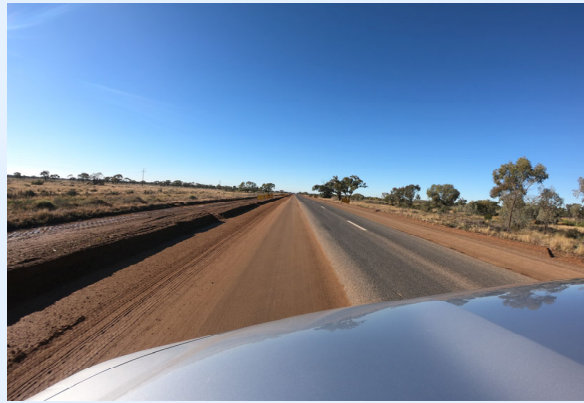
Mitchell Highway construction on behalf of the RMS
