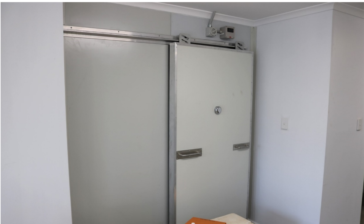
Bar Cool Room Rear – Photograph B
