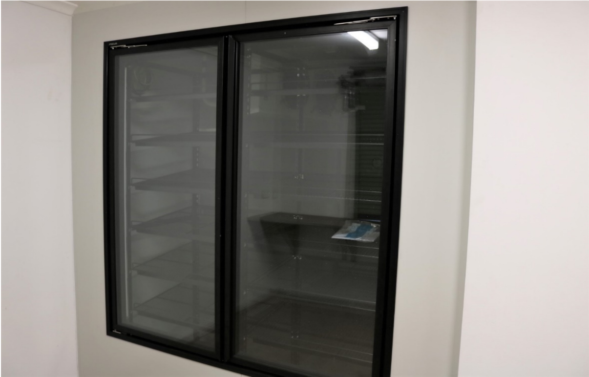
Bar Cool Room Front – Photograph A
