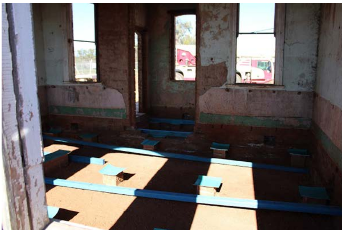
Main building waiting room construction of sub-floor timbers
