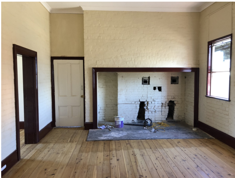
Downstairs room after
