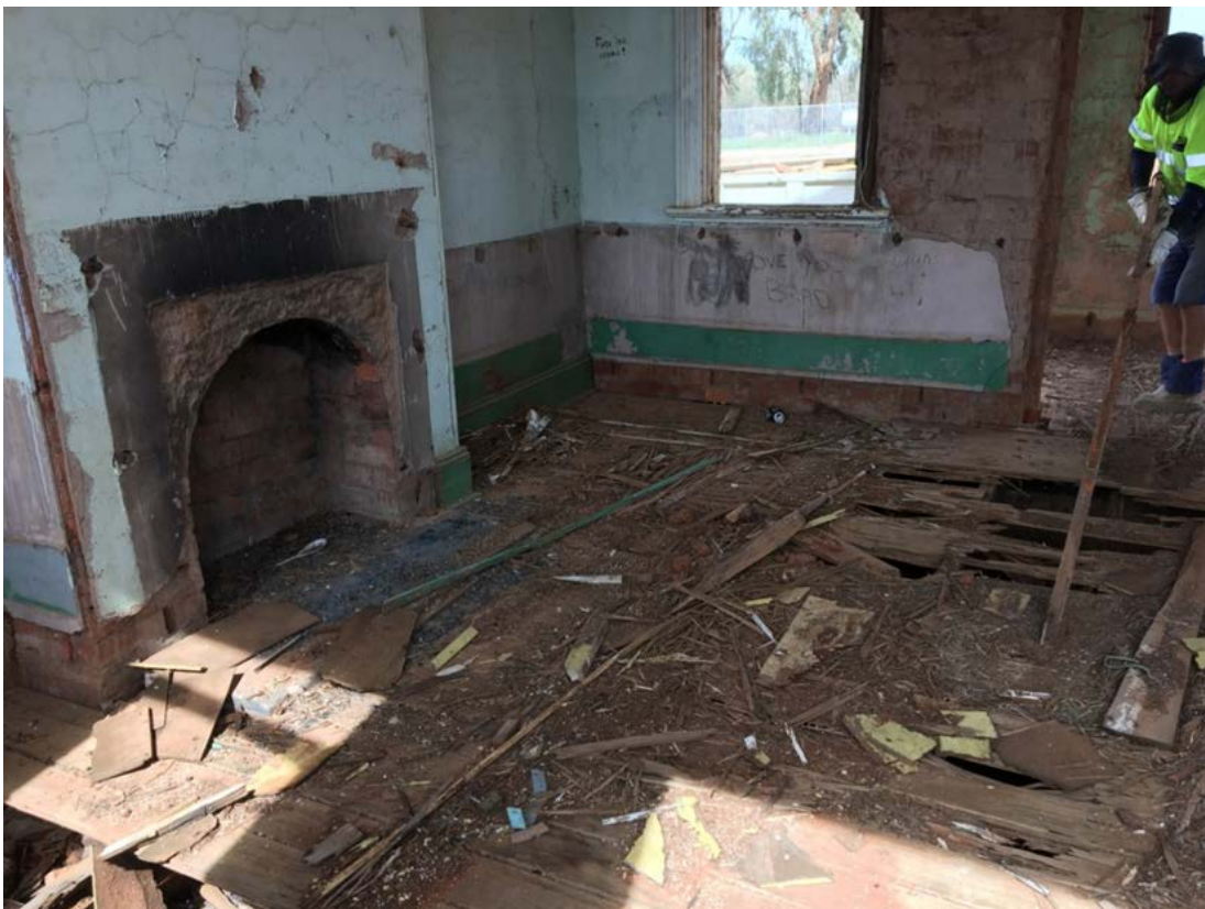
Main building waiting room before
