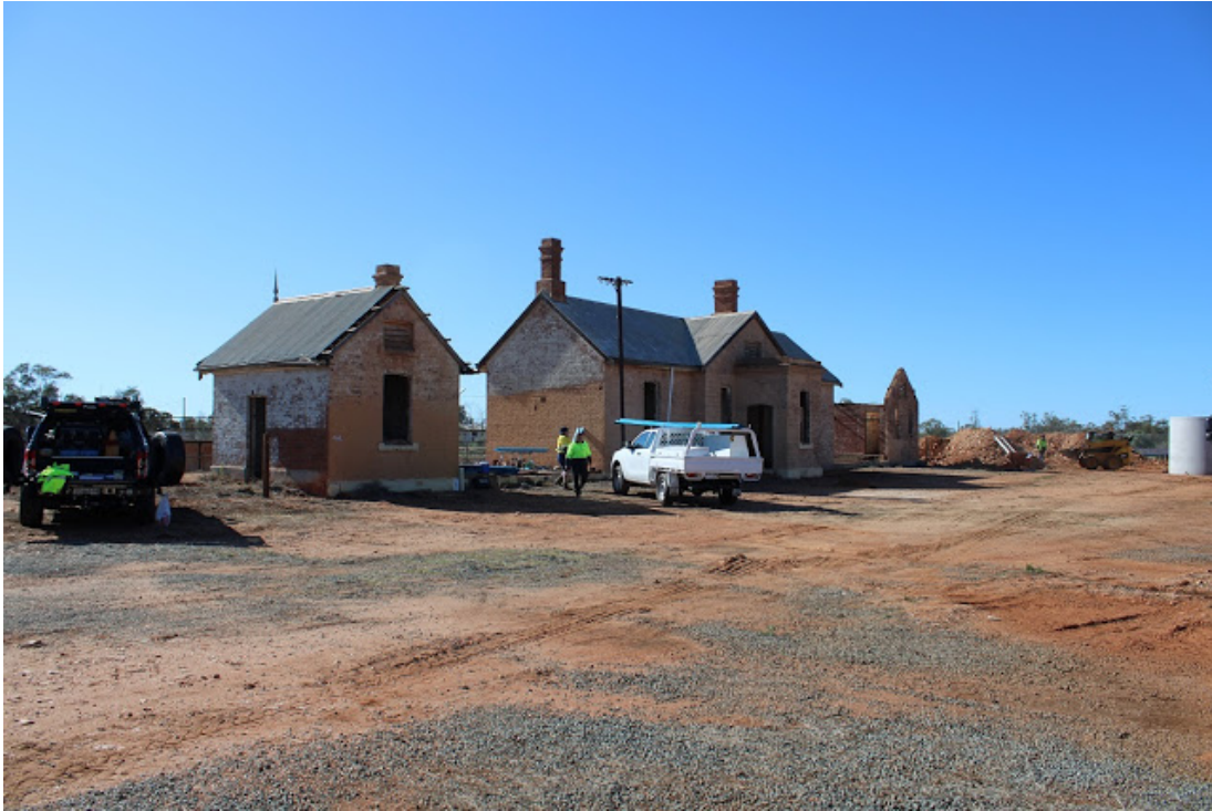
Commencement of works
