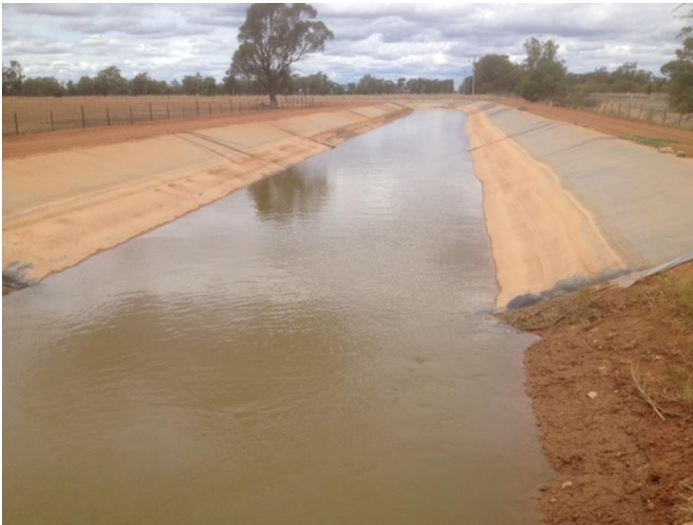
Figure 11 – Example of a channel liner near Trangie. Full fencing is essential
