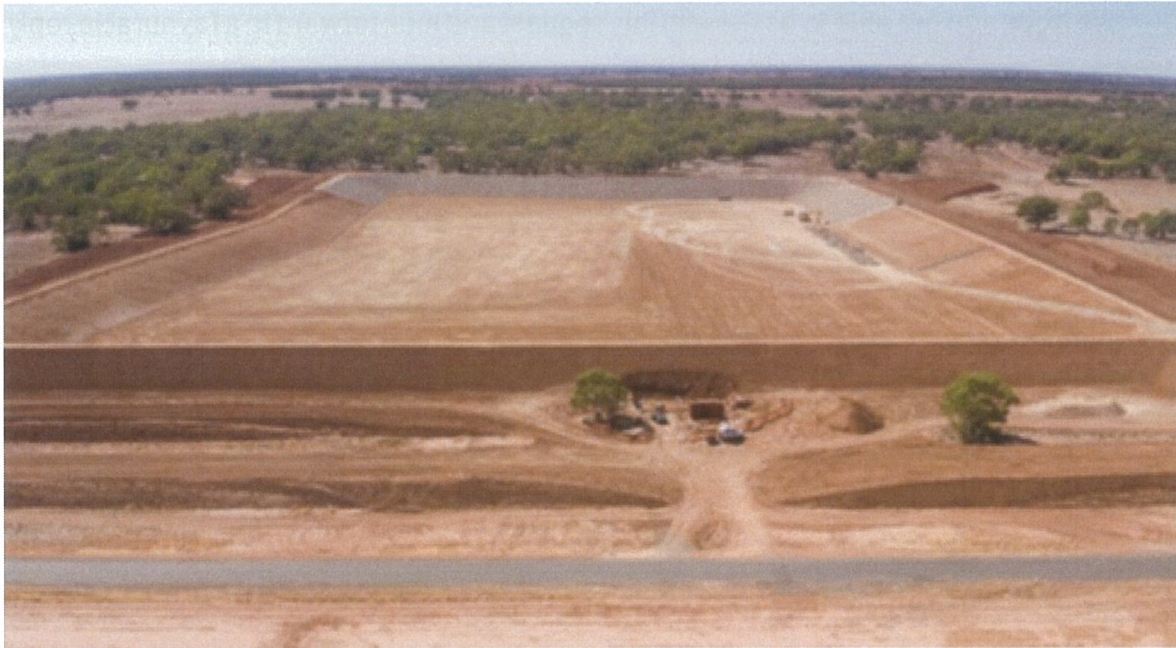
Storage Dam after completion of earthworks
