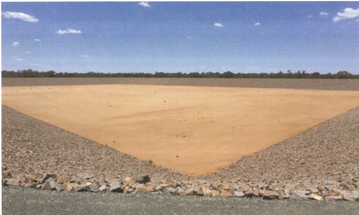
Completed storage dam
