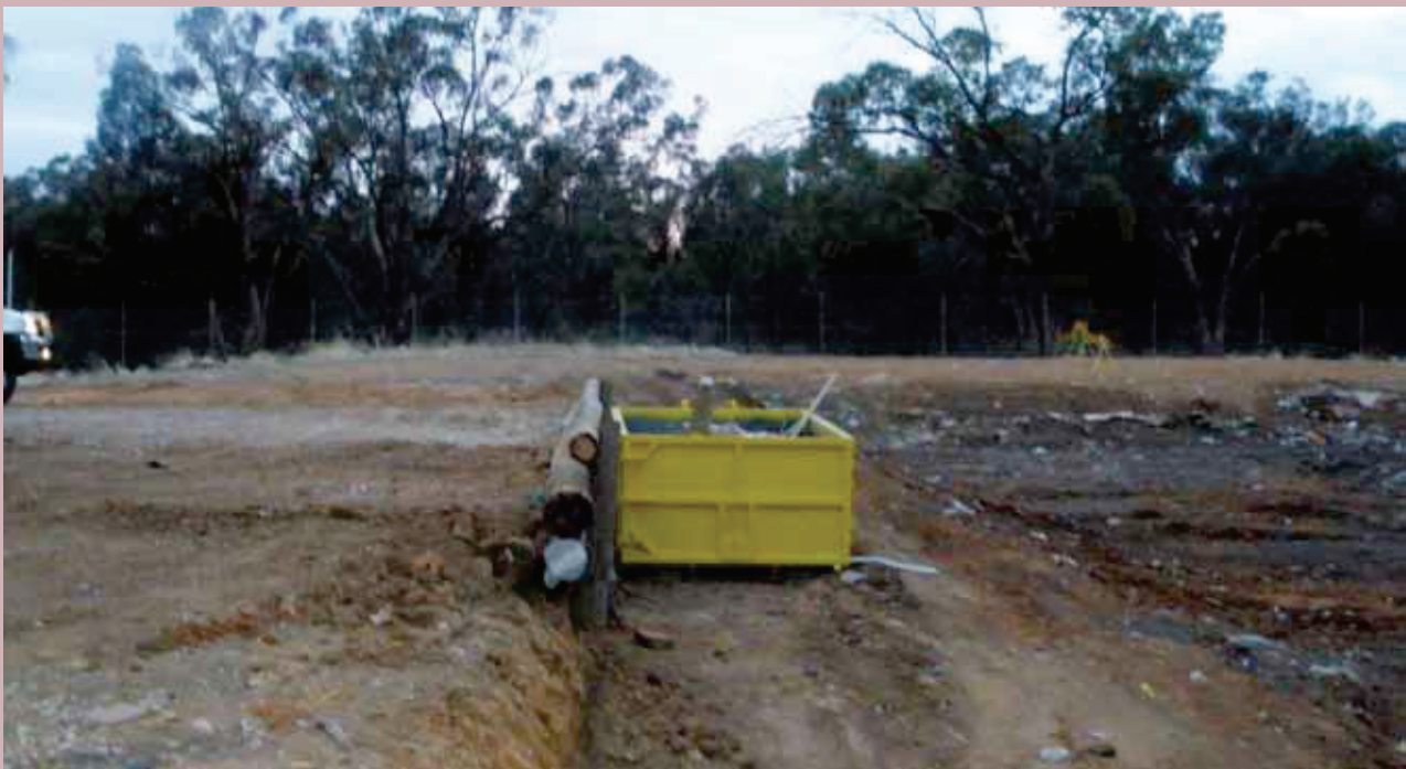
Derriwong transfer station collection point
