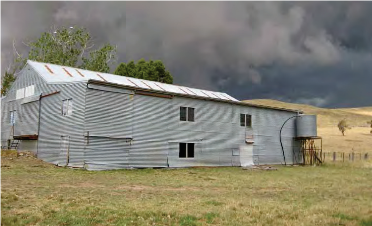
ABOVE Farm structures in Blayney
