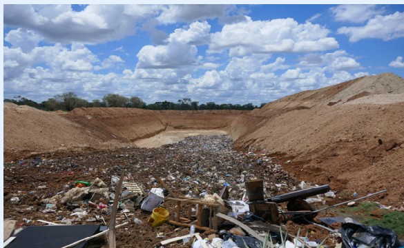
New landfill cells have been constructed at the Facility
