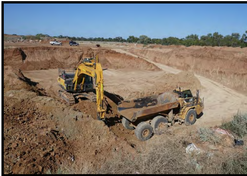
Construction of a new waste cell.
