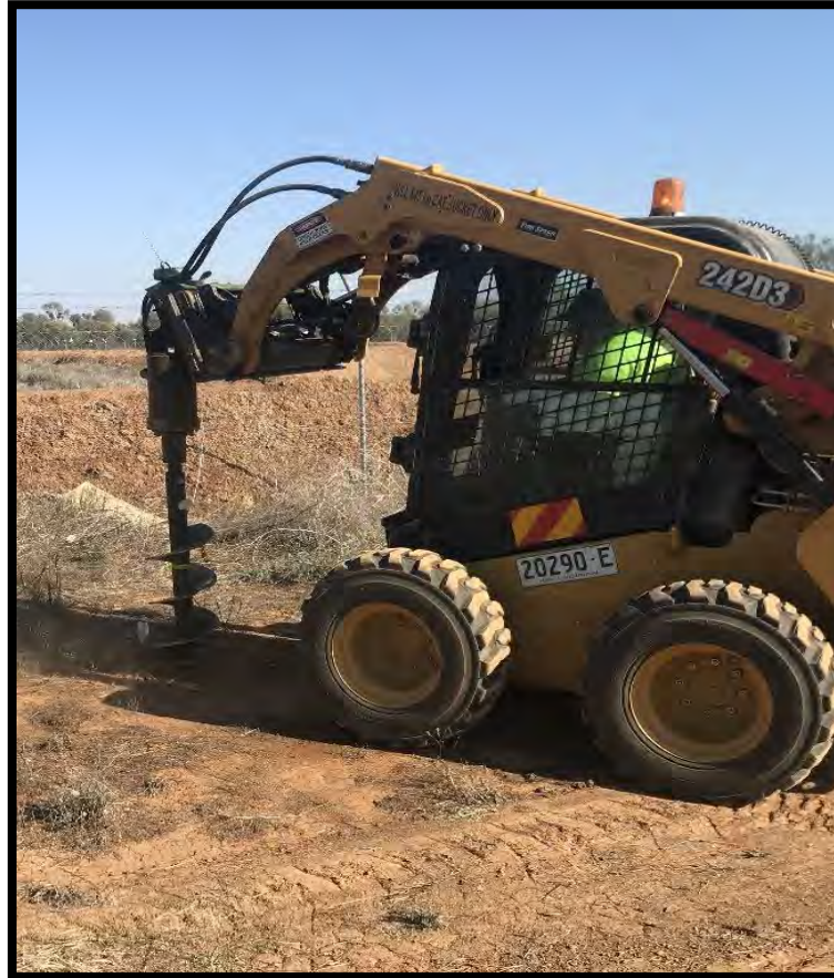
Site preparation for the planting of trees along the perimeter fence.
