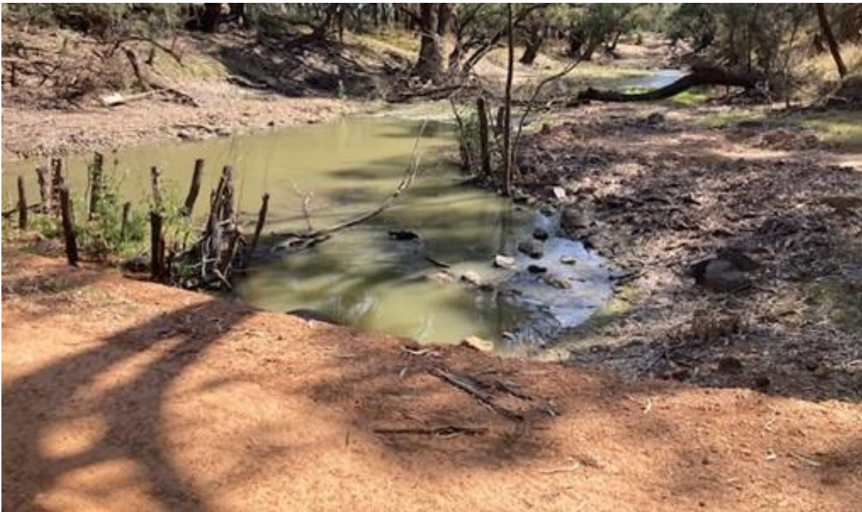
Monkey Bridge bypass looking downstream.
