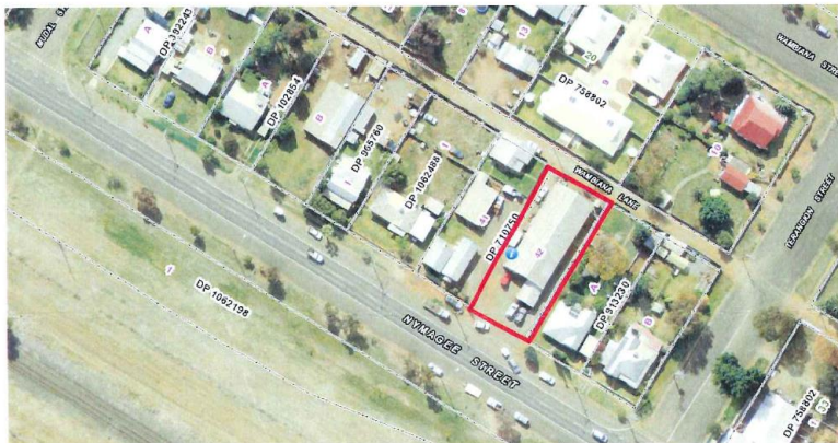
Figure 1: Aerial view of the site outlined in red (Source: sixmaps.nsw.gov.au)
