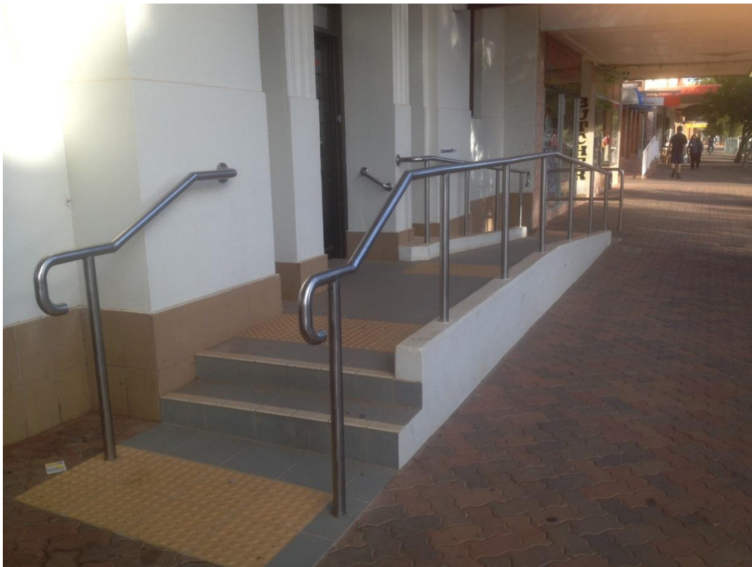
Access ramp located outside of the Commonwealth Bank of Australia
