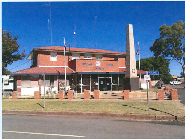
The Bogan Shire Council Chambers building at 81 Cobar Street, Nyngan.
