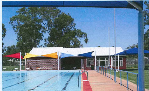
The Nyngan Swimming Pool has a new filtration plant, shade shelters and a club house.
