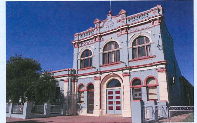
The Nyngan Town Hall was recently repainted.
