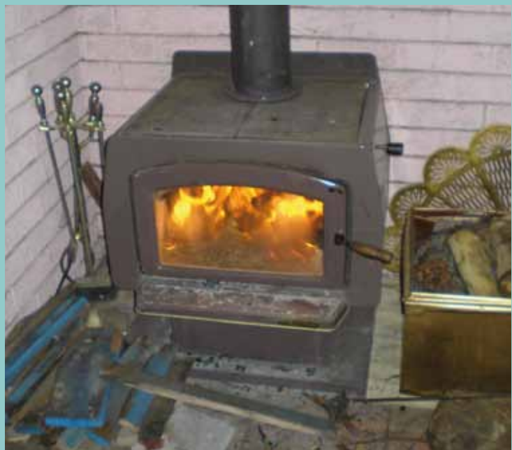
A typical older style woodheater which is often responsible for woodsmoke complaints.
